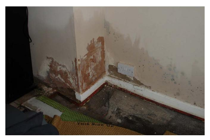
Figure 4: Elevated moisture in a wall (image © PCA)
