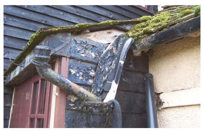
Figure 5: Defective rainwater gutters and downpipes (image © PCA)
