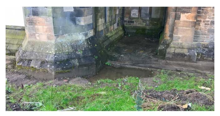
Figure 3: Defective rainwater disposal (image © Historic Environment Scotland)
