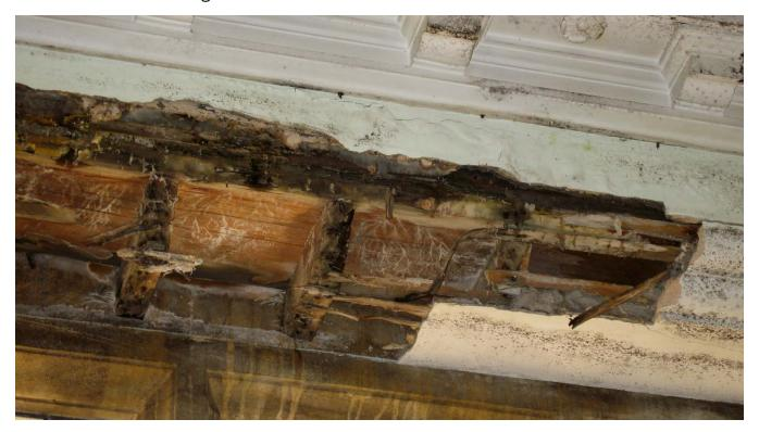
Figure 8: Collapsed plaster due to water penetration via lead parapet gutter (image © Historic England)
