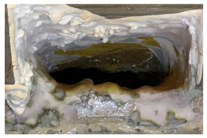
Figure 6: Dry rot under a suspended timber floor (image © RICS)
